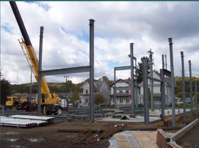
The new facility being built in Meadville, PA
