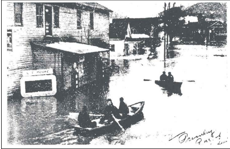
February 1945 flooding as result of ice gorge at East Hickory. (Photo from Flood Plain Information Allegheny River )
